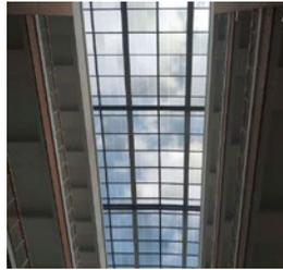
Bipv glass, CDTE cells, light transmittance 50%. Solar innova
